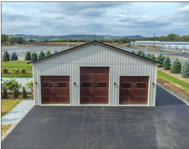
Drone image of completed pole barn garage courtesy of Extreme Pole Buildings.
