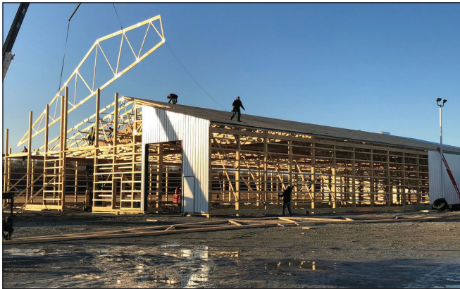
Project build in progress courtesy of CMT Components.
