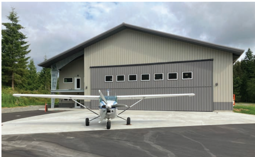
Living in an airpark is the utmost in convenience for pilots. It allows them to taxi to and from the runway right from the hangar in their home.
