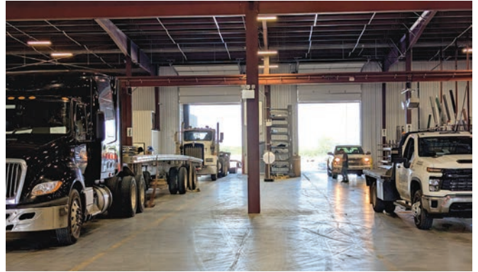
Having two lines of traffic speeds movement of material through the new facility. PHOTO COURTESY OF METAL PANELS, INC.
