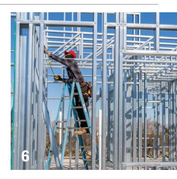
On the cover: A worker connecting components for a coldformed steel frame structure. PHOTO COURTESY OF FRAMECAD
