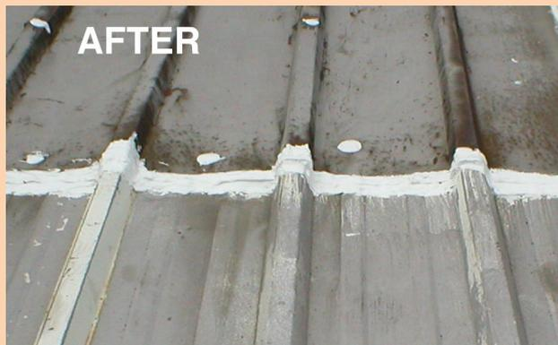
**A severe horizontal seam, before and after application of Drop-Stop®.**
