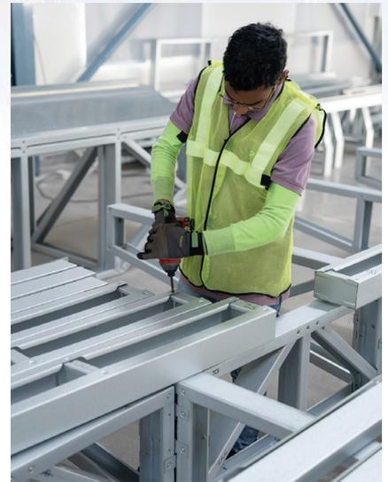
MEP systems. CFS webbed joists can be designed at standard or non-standard heights and have complex profiles for recessed floor sections. CFS joists are dimensionally stable and can accommodate various floor spans and loads.
