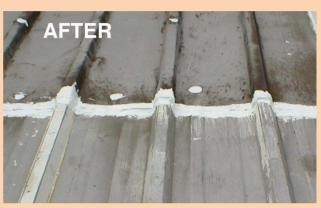
A severe horizontal seam, before and after application of Drop-Stop®. PHOTOS COURTESY OF DYNAMIC FASTENER.
