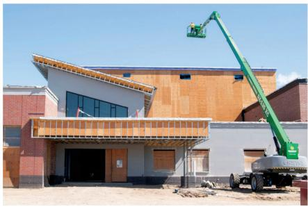
An InSpire Solar Air Heating Collector from ATAS International was installed on The Hamilton Ridge School in Minnesota. Top: Construction in progress. The south-facing wall on which the transpired solar collector will be installed. Top: Note the duct intakes through which the solar-warmed air is drawn into the ventilation system. InSpire can be installed over any non-combustible wall material. PHOTO CREDIT: ATAS INTERNATIONAL
