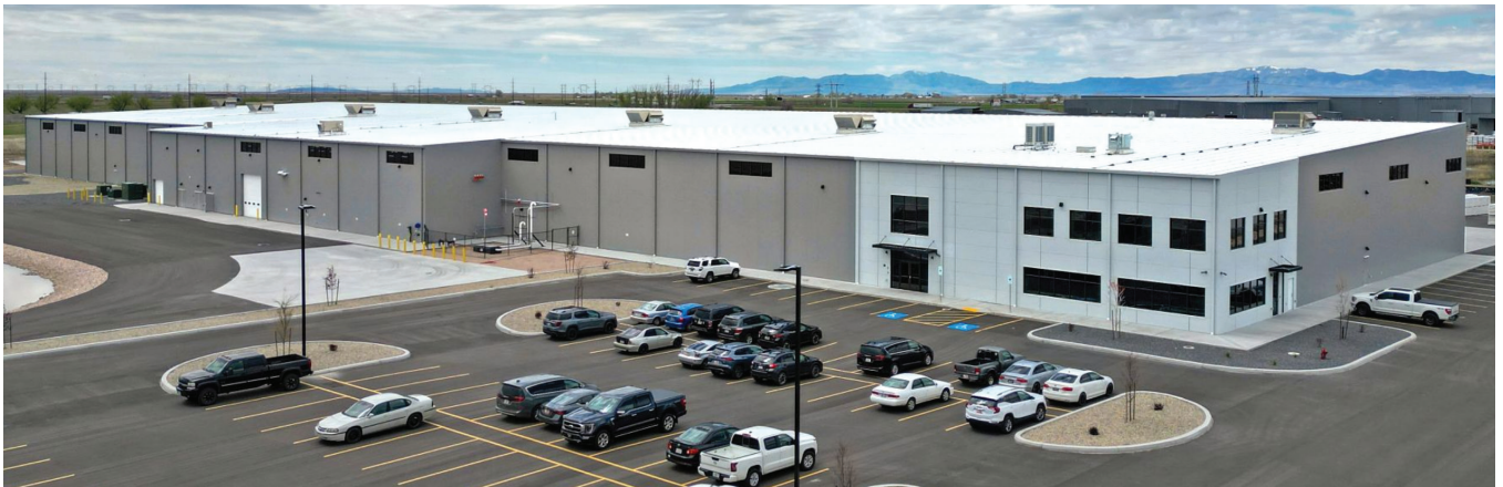
Nucor's new Metl-Span Manufacturing Facility in Utah.
