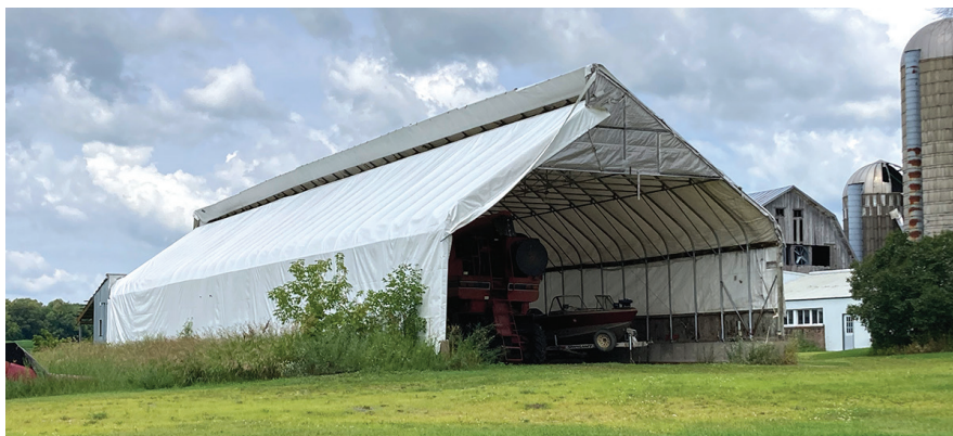
Even an older combine can be worth hundreds of thousands of dollars. A steel-frame tension fabric building can be a cost-effective way for a farmer to protect it from the elements.
