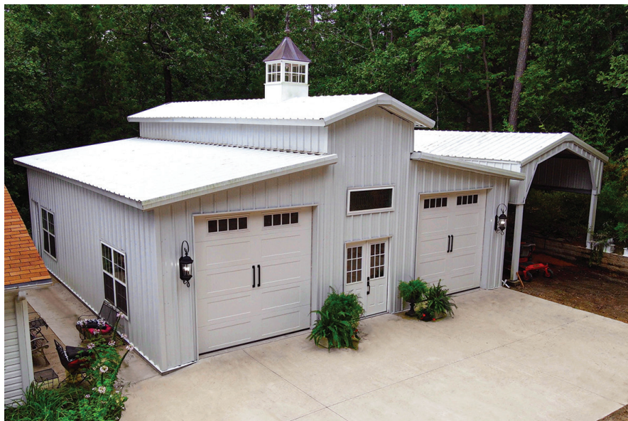
A cold-formed steel structure like this Hypersteel™ farm building has many benefits, such as ease and speed of construction; high strength-to-weight ratio; large clear span capabilities; and fire, pest, termite, and mold resistance. PHOTO COURTESY OF CORNERSTONE BUILDING BRANDS.
