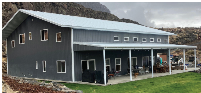
PHOTO COURTESY OF WORLDWIDE STEEL BUILDINGS
