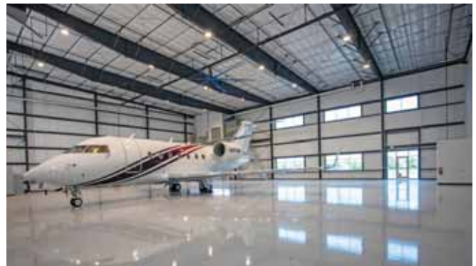
The increase in insulation requirements in the IECC has made the most substantial contribution to building performance. PHOTOS COURTESY OF METALCON.
