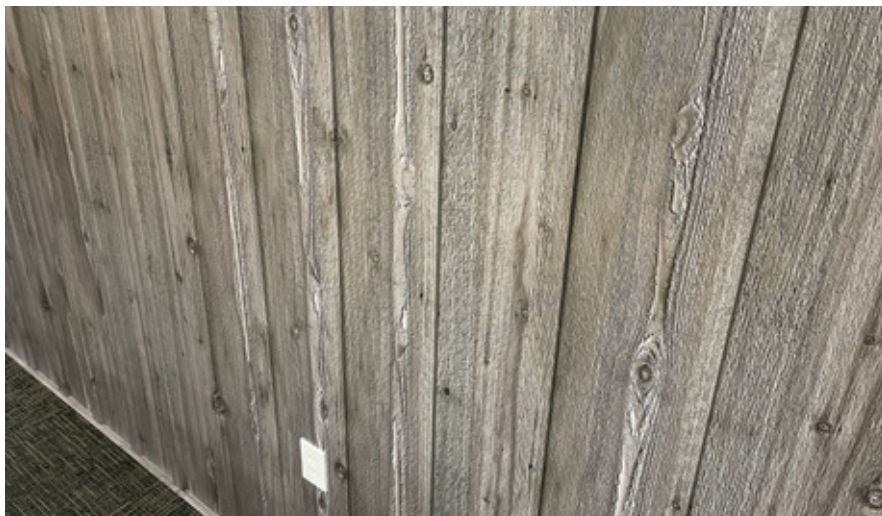
Graber Post Buildings was consulted to help develop digital prints that would appeal to the growing popularity of board and batten siding. Graber installed some of the wood, rough sawn cedar in gray, for an office conference room shown here. GRABER POST PHOTO
